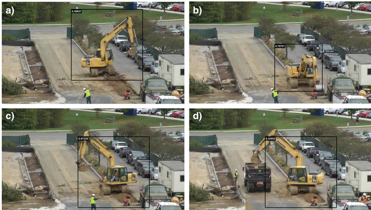
Fig. 22. Detecting an excavator in a video sequence wherein the pose is rapidly changing.
