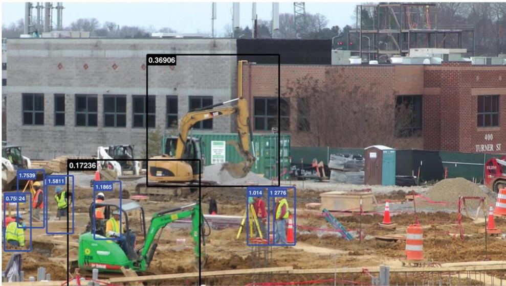
Fig. 24. Detection of excavators and construction workers in proximity of each other.
