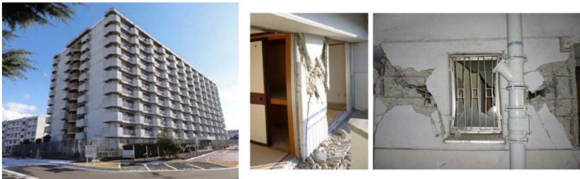
(a) Non-structural walls failed in shear
