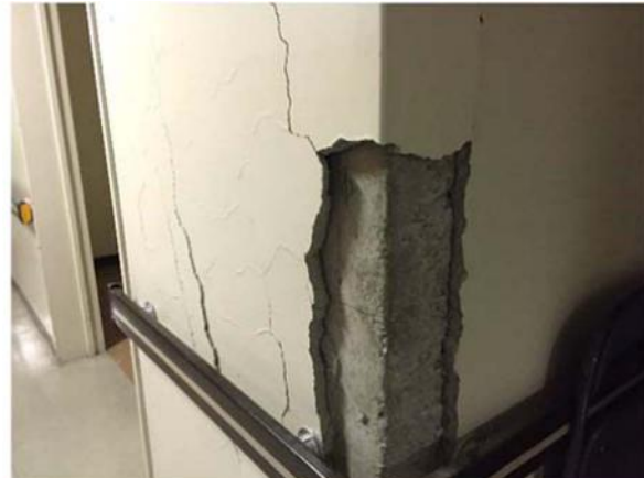
(b) Minor cracks on columns
