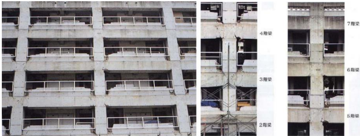
(a) Flexural cracks of beams
