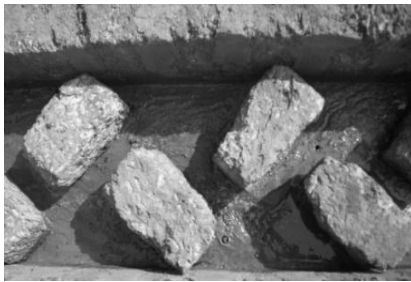
Figure 3. Inclined baffles
