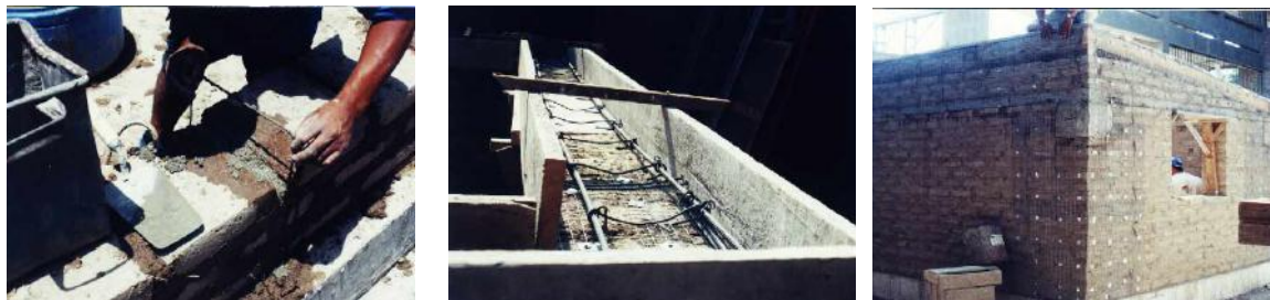
Fig. 7. Some structural improvements in the new adobe houses: wire connector in joint (left), collar beam (middle), and shear key (right).
