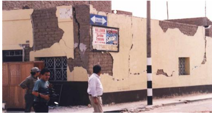
Fig. 2. Typical cracks on adobe houses due to out-of-plane seismic forces.
