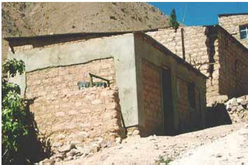
Fig.5. Reinforced house and unreinforced neighbor houses after the 2001 earthquake.
