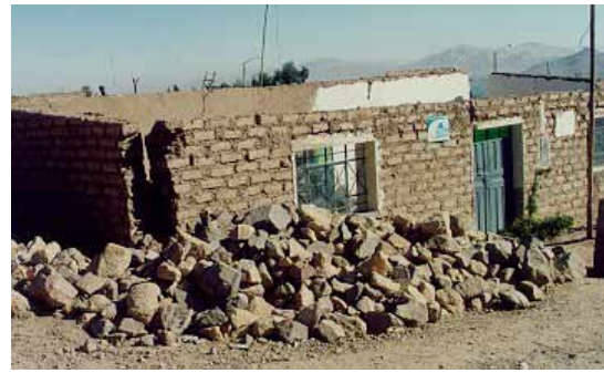
Fig.5. Reinforced house and unreinforced neighbor houses after the 2001 earthquake.
