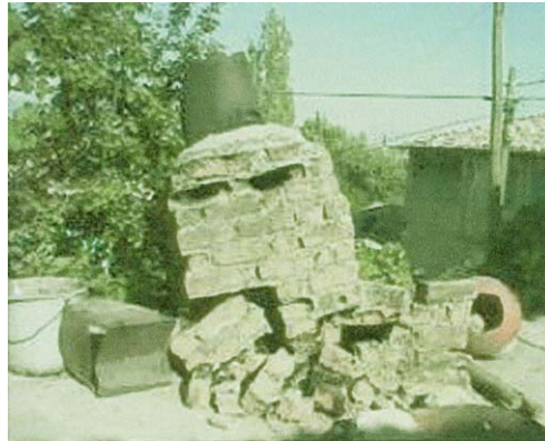
Fig. 17. A collapsed chimney of traditional building during the 2003 Buldan earthquake [15].
