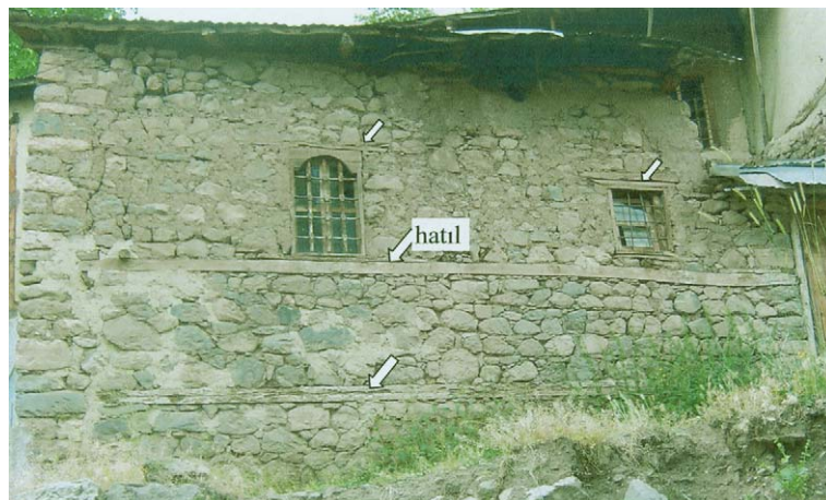
Fig. 4. Traditional hatıl construction in Turkey.
