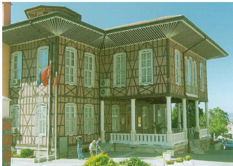
Fig. 5. Traditional hıms building with bracing elements and brick infill in Bursa.
