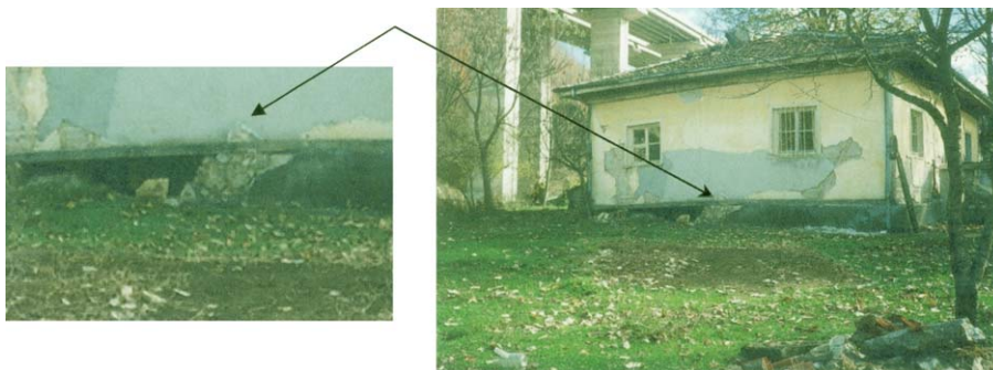
Fig. 16. Failure of masonry foundation of a himiş construction just over the fault rupture during the 1999 Kocaeli earthquake.
