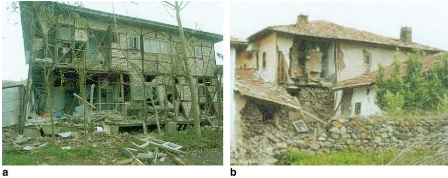
Fig. 14. Masonry falling out of the frames for traditional himiş constructions. (a) Damaged during 1999 Kocaeli earthquake [7]. (b) Damaged during 2000 Çankırı earthquake [19].
