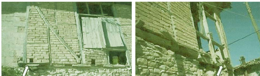
Fig. 15. Slide off frame elements from supporting systems during the 2003 Buldan earthquake [15].
