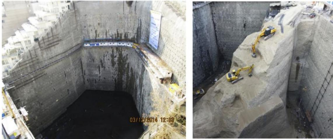
Fig. 1. A very deep excavation in the northern part of Tehran with the maximum depth of 70 m.
